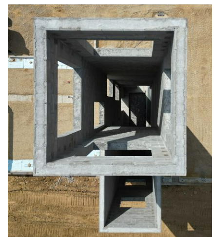
Peering down the newly constructed bell tower eagerly awaiting bells
